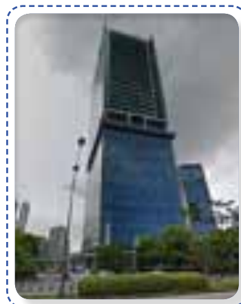
Cyber 2 Tower Green Building Gold Rank (81 points) / Peringkat Green Building Gold (Poin 81) Year 2007-2009 / Tahun Pelaksanaan 2007-2009
